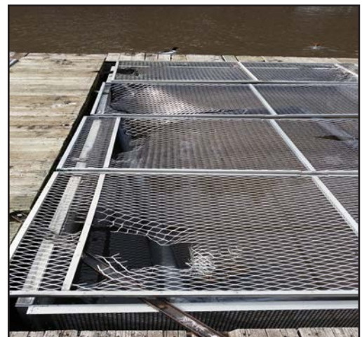
Cage covers damaged by River Otters.
